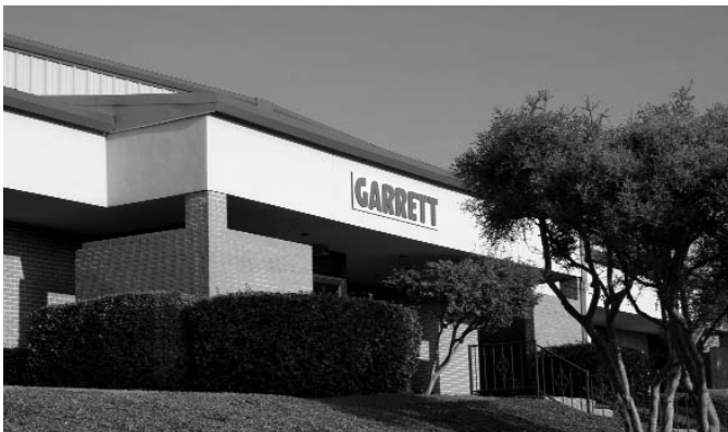
Garrett's current headquarters which includes manufacturing facilities and the company's engineering laboratories will be significantly expanded to meet growing customer demands.
