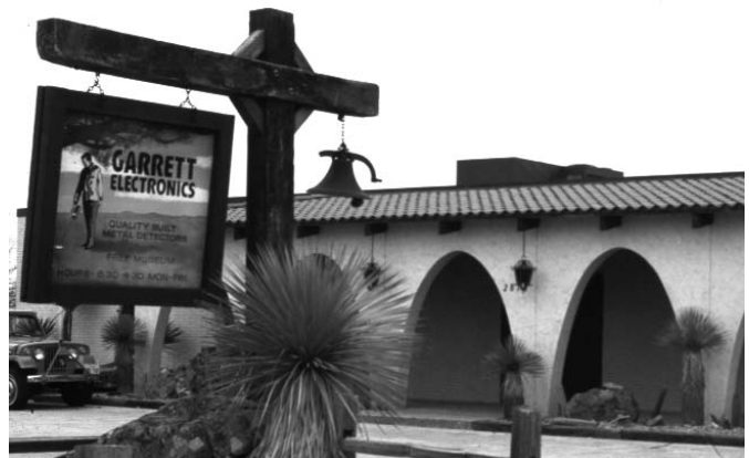
With architectural design in the spirit of the Old West, Garrett's first major facility contained its offices, showroom and manufacturing operations and was constructed in 1970 on National Drive in Garland.
